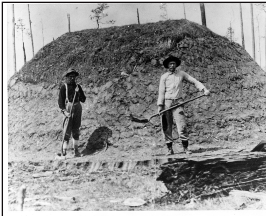
Charcoal pit at Gainesville, Mississippi, on the Pearl River in Hancock County in 1912. The two charcoal burners are shoveling dirt onto the pit. Photograph courtesy of the Hancock County Historical Society.
