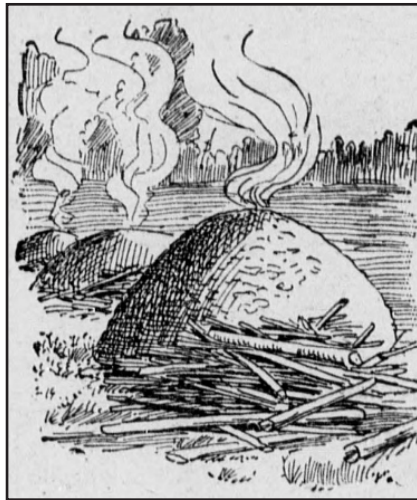
Burning charcoal pits, most always called charcoal or coal kilns in Mississippi, and usually constructed in groups of six to ten so that the charcoal burner could supervise multiple charcoal pits simultaneously. From Scranton Chronicle, January 30, 1904.
